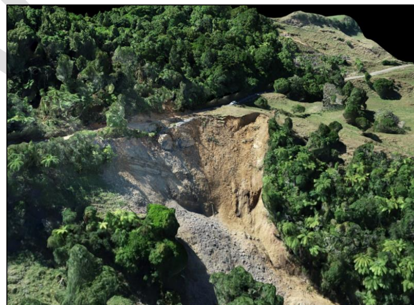
Figure 15: Taumatotara West Road, one of the worst effected roads resulting from Cyclone Dovi (2022)
